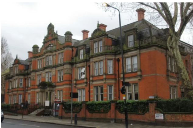
The Register Office, 317 Harrow Road W9 3RJ
